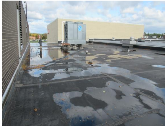
Partial Overview of Roof Area 7
