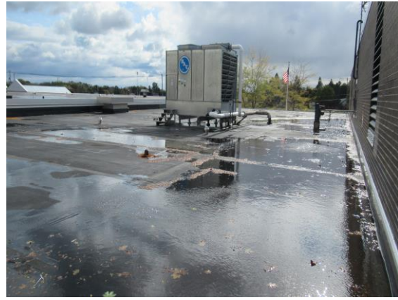
Partial Overview of Roof Area 7
